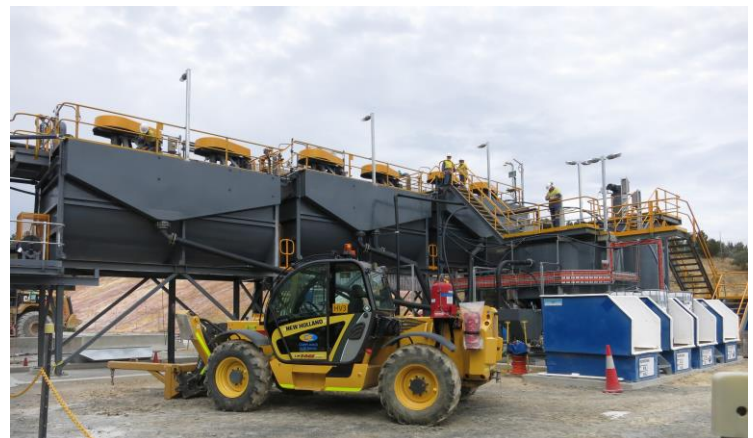
Left image 3Q2015: Flotation cells lifted into position in the flotation circuit. Bottom image 4Q2015: Progression of the addition of flotation circuit and ball mill.
