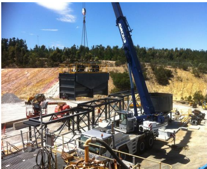
Left image 3Q2015: Flotation cells lifted into position in the flotation circuit. Bottom image 4Q2015: Progression of the addition of flotation circuit and ball mill.
