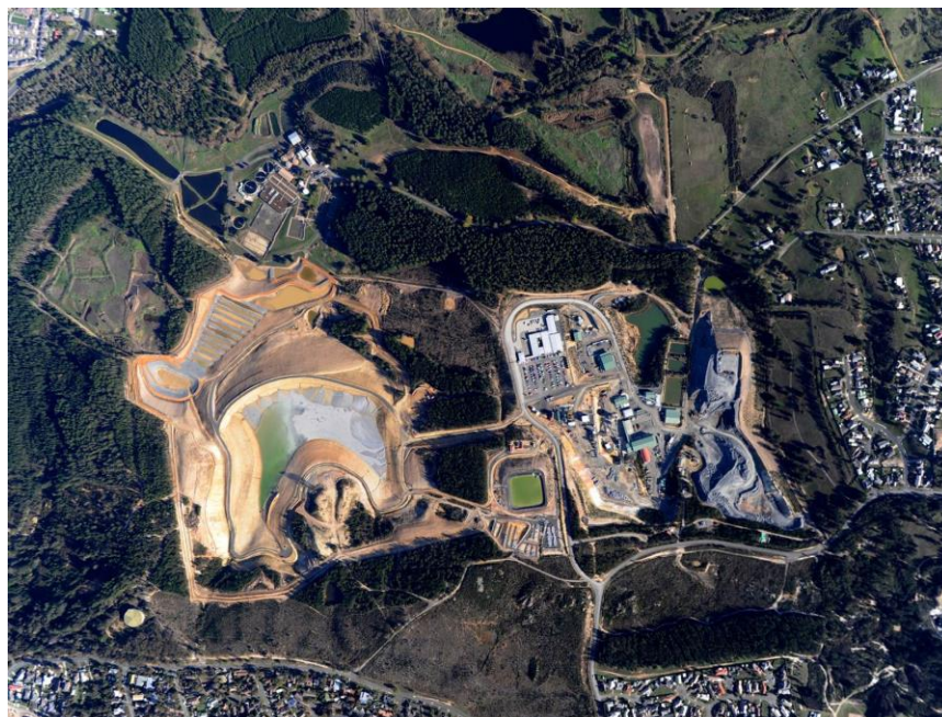
Aerial view of Castlemaine Goldfields' Ballarat Mine
